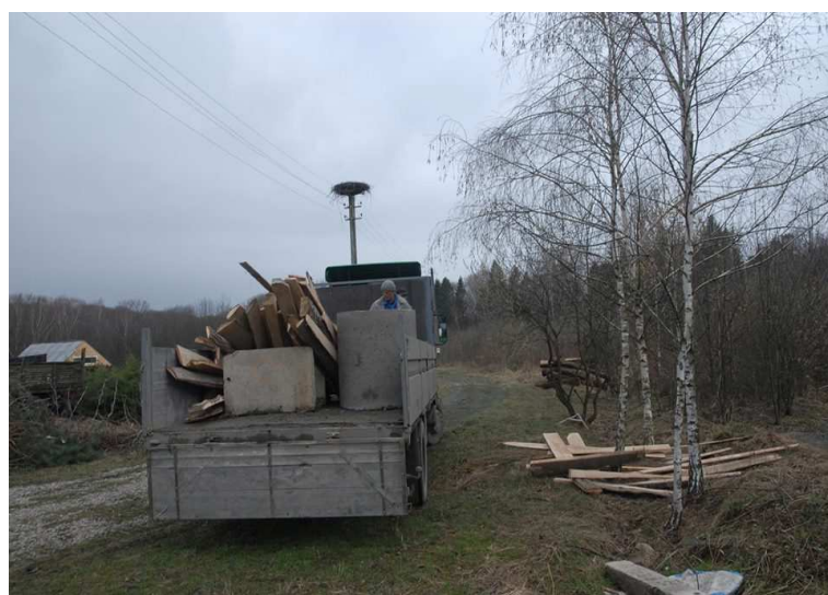
Unloading materials to build enrichment facilities – Photo courtesy of Eco-Halych
